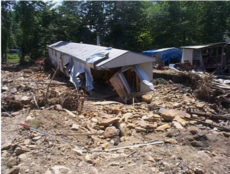
Figure 1-4. Example of Flood Damages in July 2001
