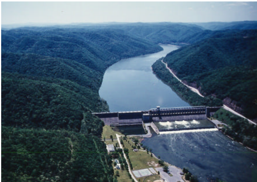
Figure 4-4 Bluestone Dam in Summers County, West Virginia
