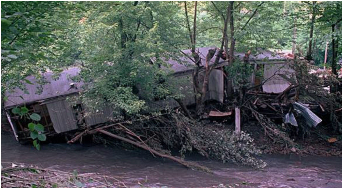
Figure 6-1. Inadequately Secured Manufactured Home Following A Flood
