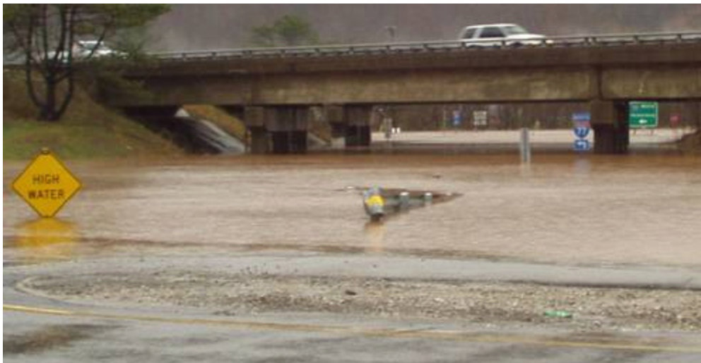
Figure 6-2. Roadway under Interstate 77 blocked by high water during a major flood event
