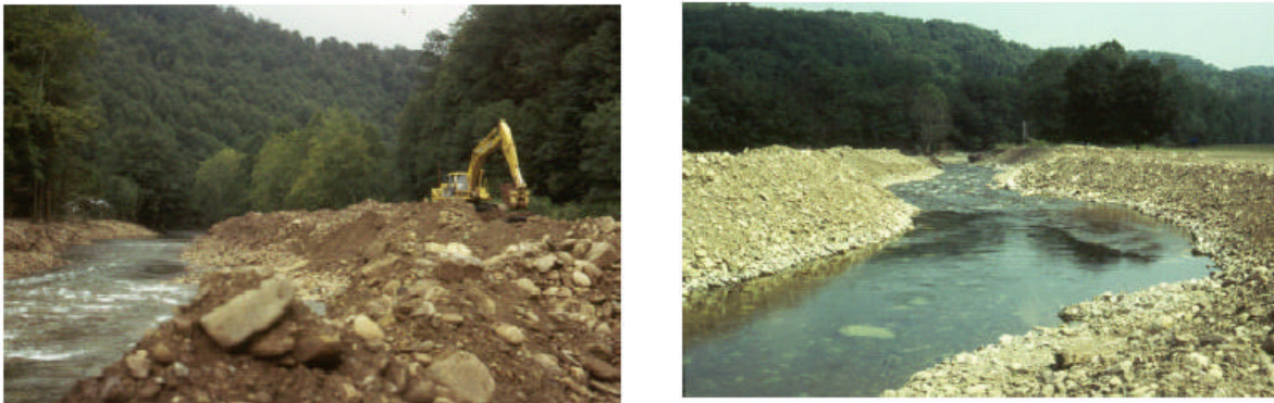
Figure H-3. Dredging of a small stream
