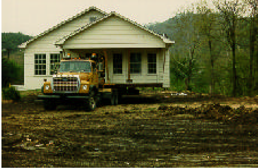
Figure L-9. Residential structure being relocated from floodway.
