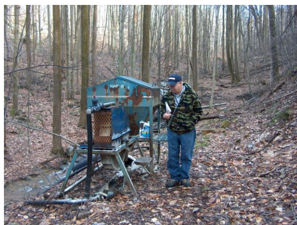
Leroy Stanley inspected a water-wheel lime doser device to determine if it is treating acidity that might pollute the Tygart River watershed.
