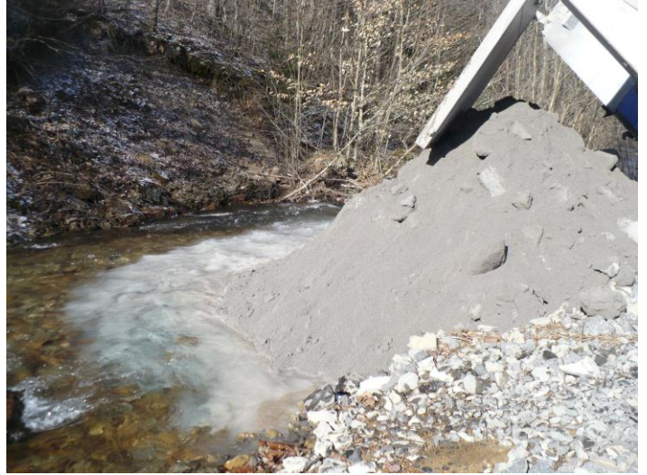
Limestone sand was poured downstream to neutralize the acid so that trout could survive in Taylor Fork.
