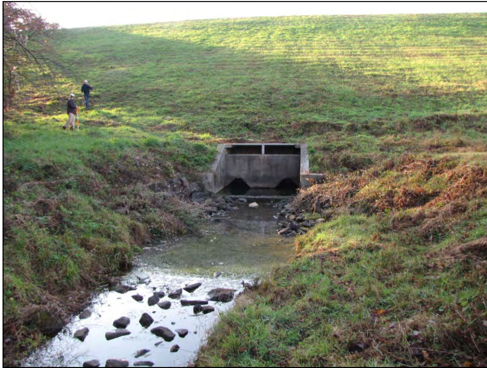
5. Outlet channel and stilling basin.
