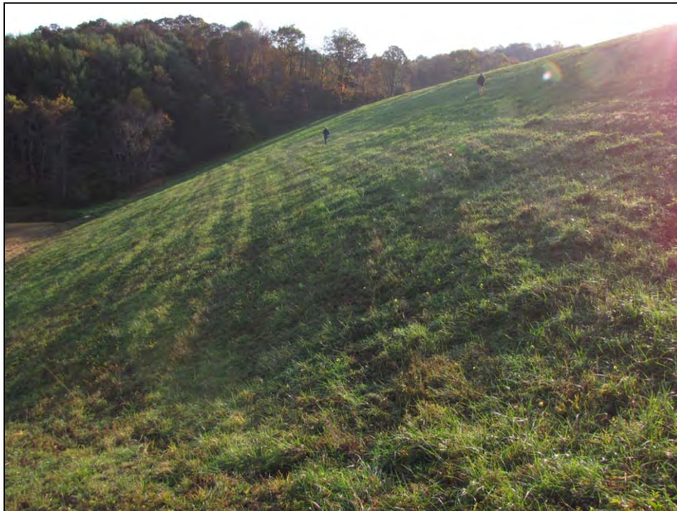
4. Downstream embankment slope.
