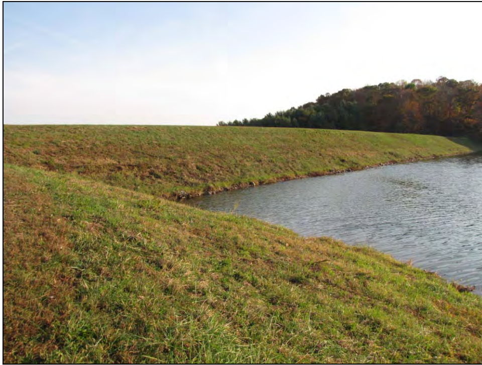
3. Upstream embankment slope.
