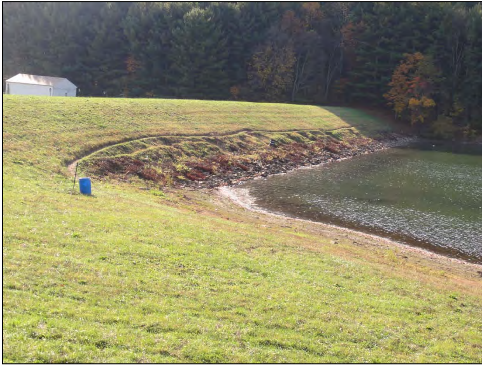
3. Upstream embankment slope.
