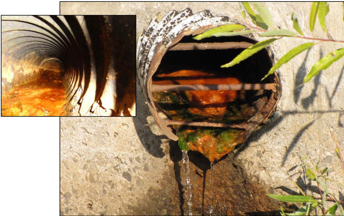
15. Left CMP drain.
