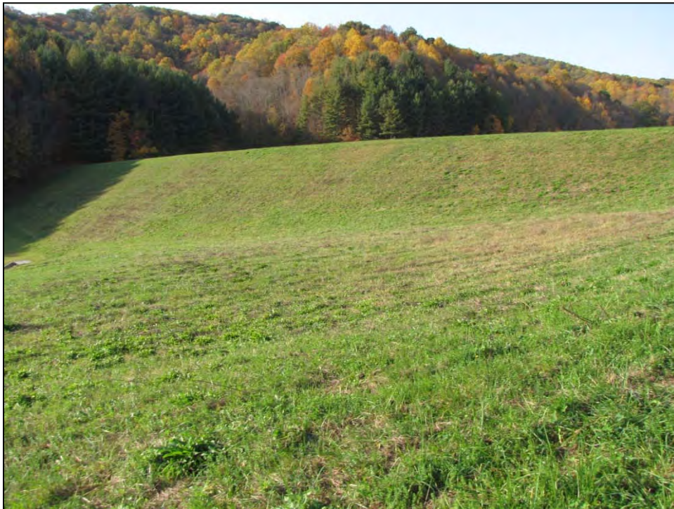
4. Downstream embankment slope.
