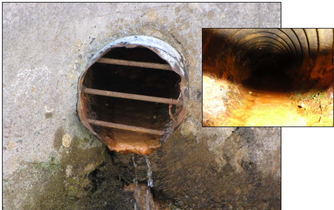
16. Right CMP drain.
