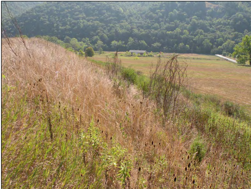
4. Downstream embankment slope.
