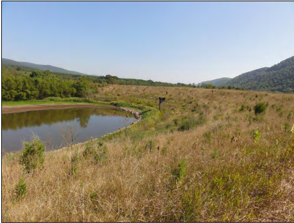
3. Upstream embankment slope.
