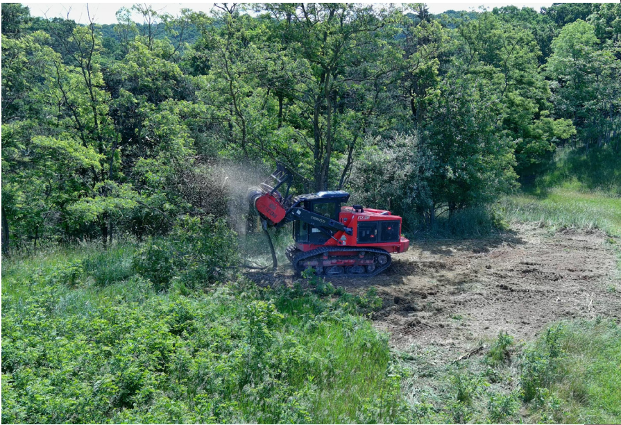
Top left: A forestry mulcher was used at Patterson Creek No. 30 dam in Mineral County to help reclaim the dam's footprint. Top right: The riser and embankment on a snowy day at Brush Creek No. 14 in Mercer County. Bottom right: A regrade of the auxiliary spillway at Patterson Creek No. 27 dam was completed in 2024.
