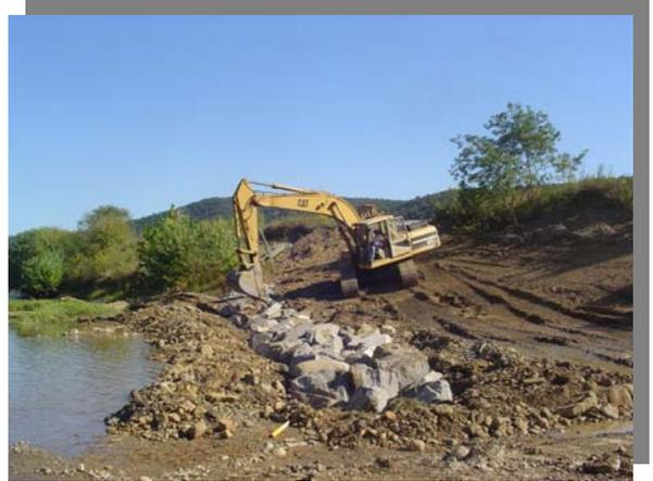
appropriate angles and slopes were adhered to and the rock was compacted into place. The idea behind building the structures in this manner was to reduce construction time and costs. Upon the end of construction, steeply eroding areas were reshaped to a 2:1 slope or flatter, reseeded, and a riparian buffer was established. Woody vegetation will be established in the Spring. Approximately 500 linear feet of stream bank was stabilized through this project.
