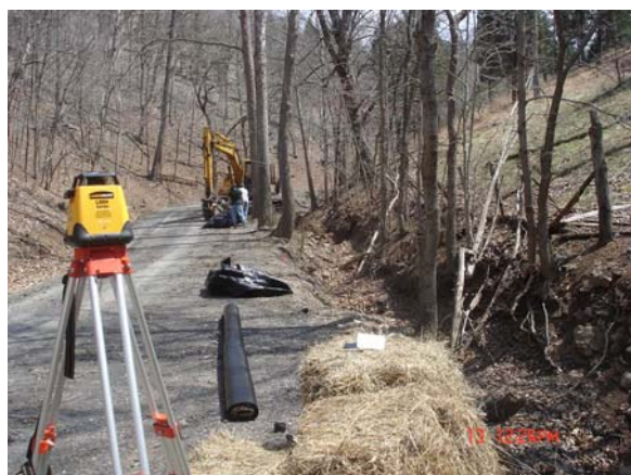
Site during construction.
