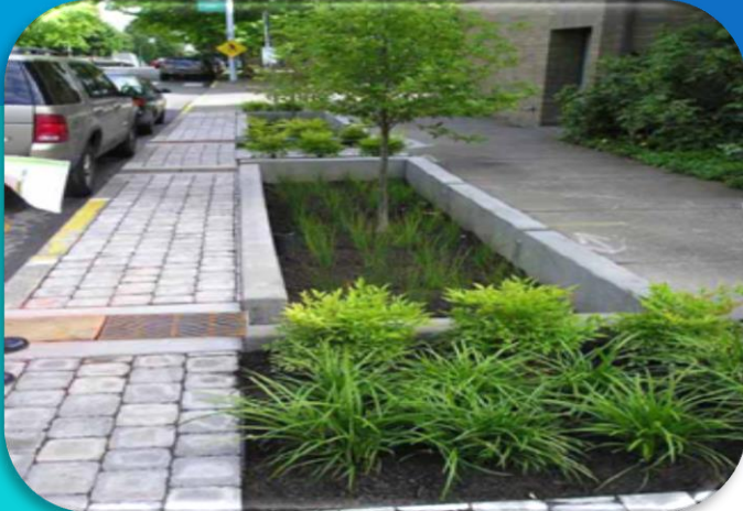
Street runoff collects in stormwater planters.
