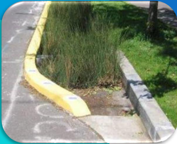
A landscaped curb extension calms traffic and captures and infiltrates street runoff.
