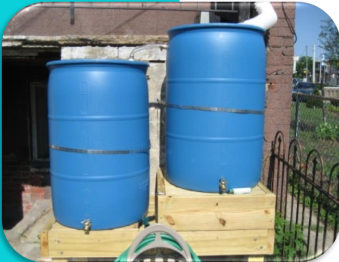
A rain barrel captures and stores roof runoff for later use.
